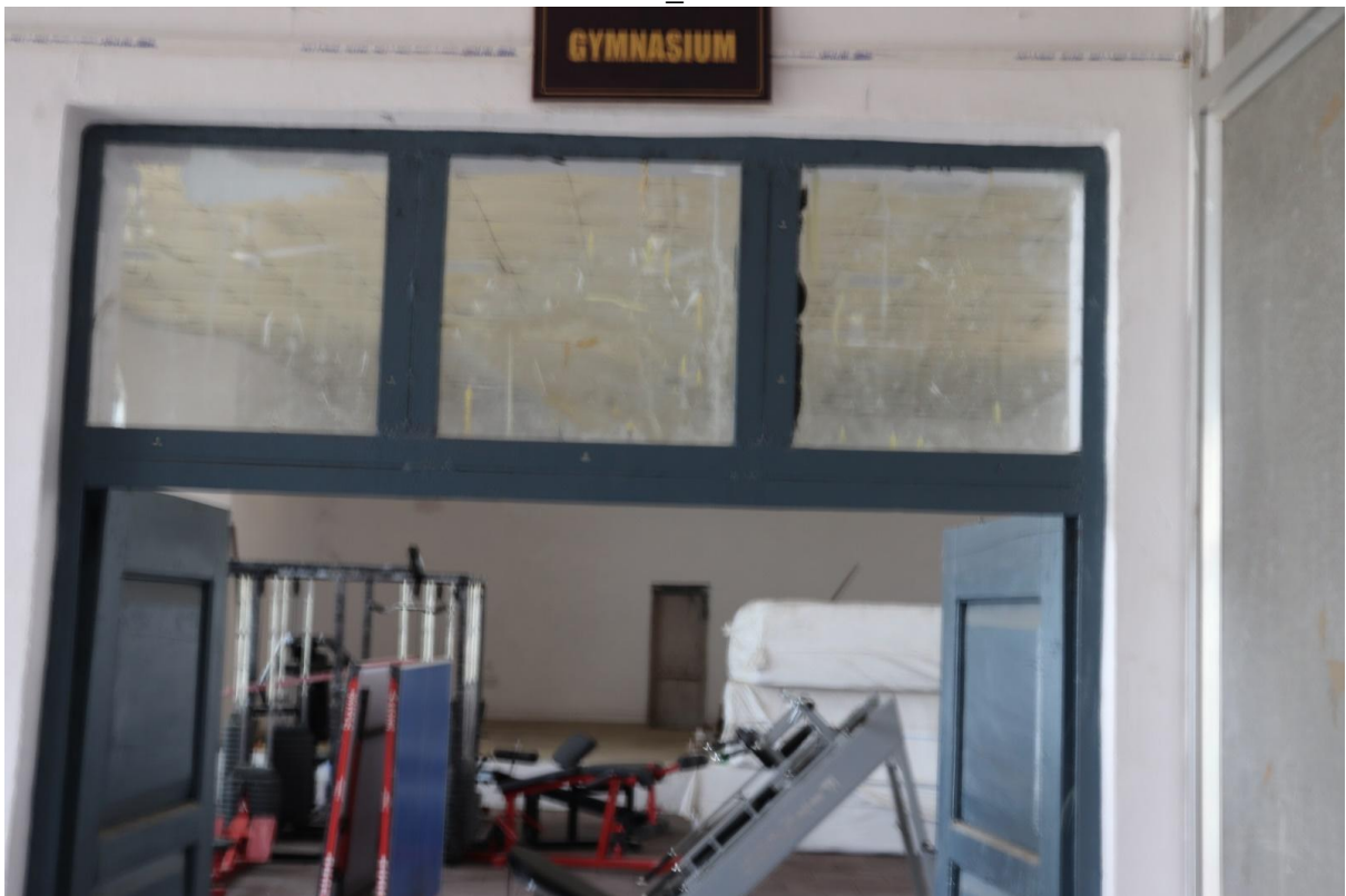
Photograph 2 Gymnasium: View from entrance
